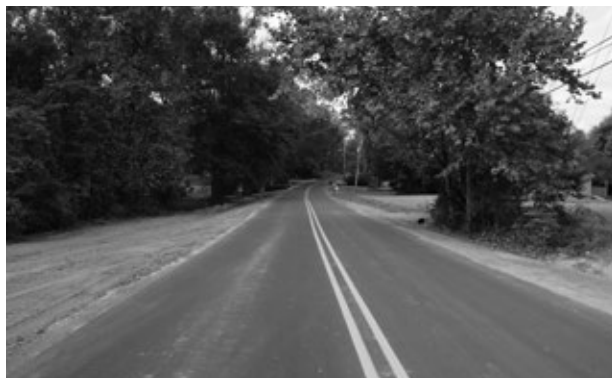
Moores Mill Road after initial resurfacing in October 2013.
